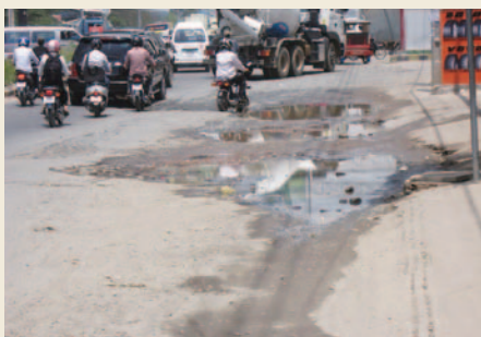
Large holes in the road surface cause traffic congestions and accidents. (Photo: IKEE Group)
